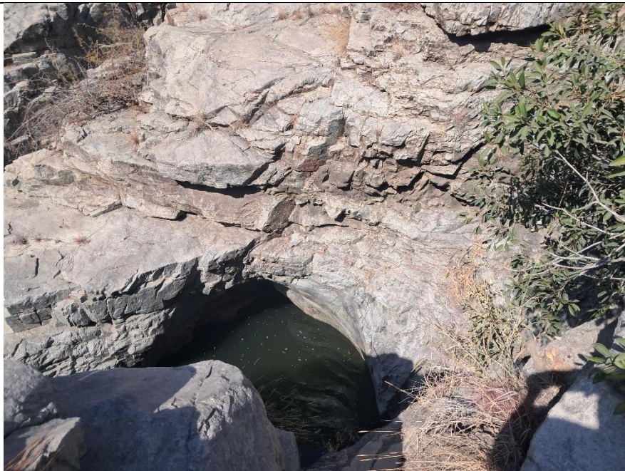
Fig 25 A large pothole in the channel at the end north end of the site.
